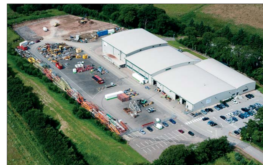
EnerMech's extensive new facilities at Howes Road in Aberdeen
